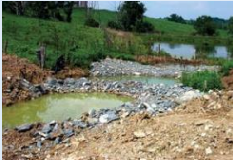
Figure 9 Examples of temporary silt traps
