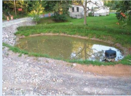
Figure 9 Examples of temporary silt traps
